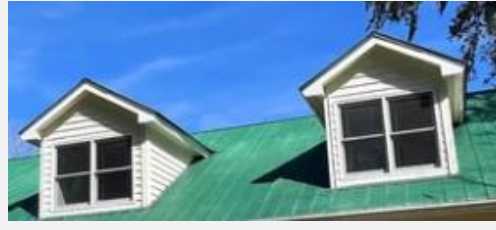
Example of oxidized roof. Before left, after right.
