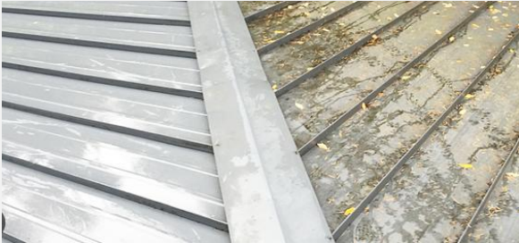
Example of regular roof service: Painted roof
